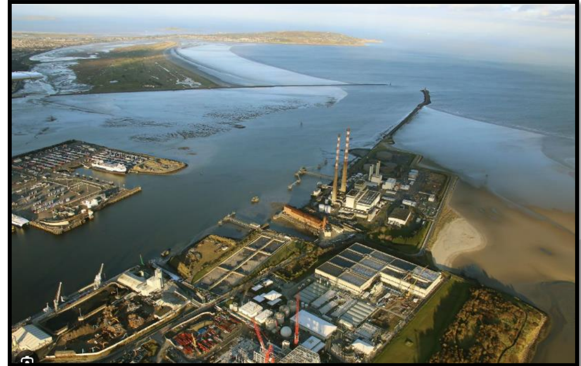
Ringsend Wastewater Treatment plants: image by Uisce Éireann
