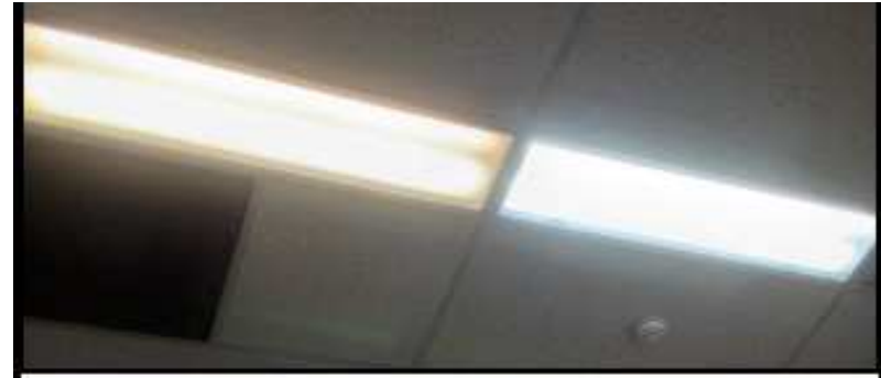
Figure 11 - Typical Twin T8 vs LED Batten 20
