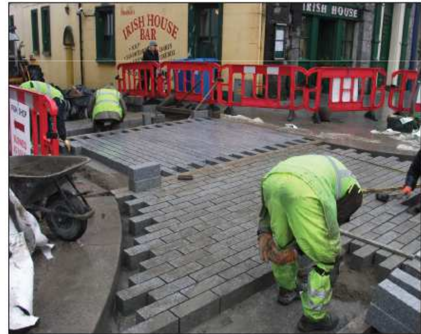
Figure 7: Ridgid Paving using granite setts bedded in mortar on concrete roadbase
