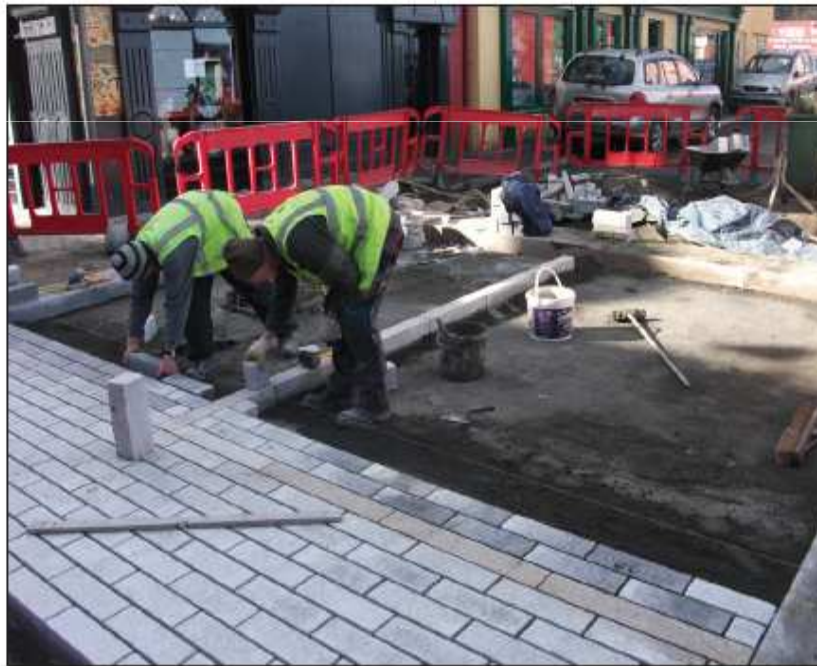
Figure 7: Ridgid Paving using granite setts bedded in mortar on concrete roadbase
