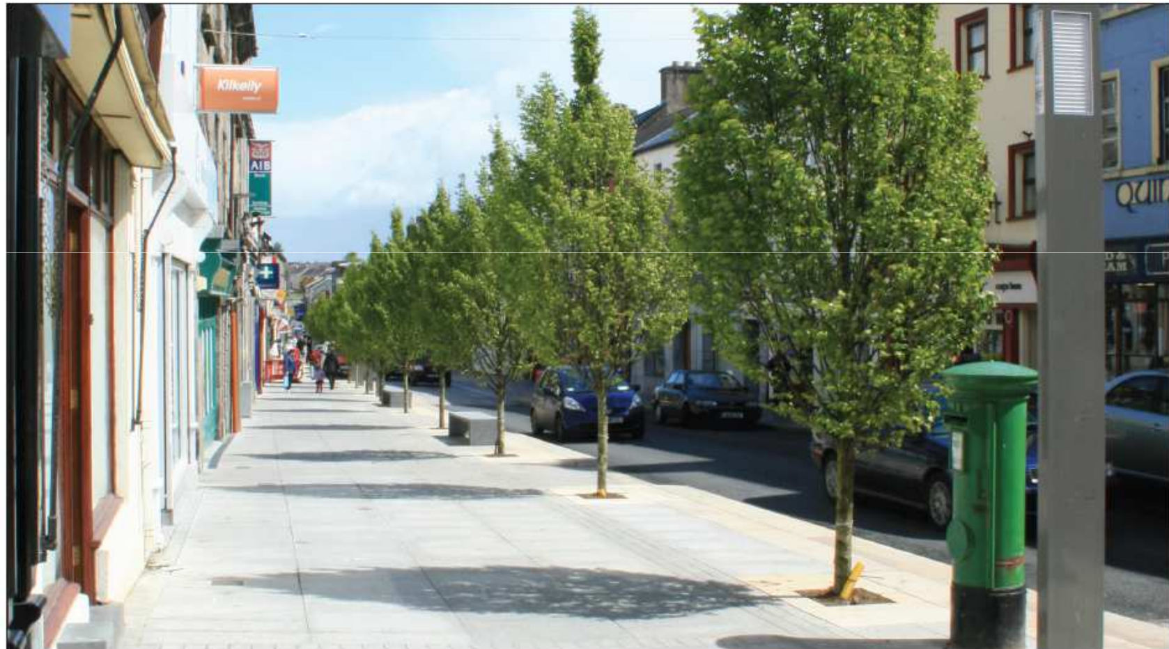
Figure 1. Well considered schemes enhance place, prioritise sustainable movement, calm traffic and provide longer term durability.
