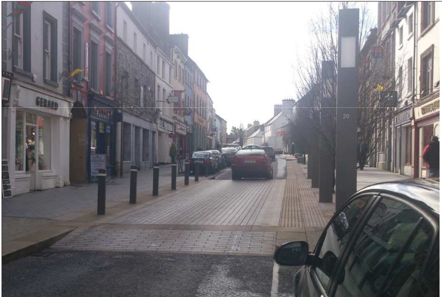
Figure 14: Completed raised table.
