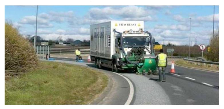
High Velocity Impact Shot Blast Providing Microtexture improvement on polished HRA
