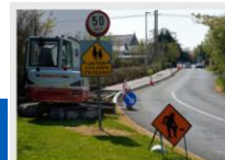
The new footpath under construction at Bennekerry. Photos: michaelorourkephotography.ie
