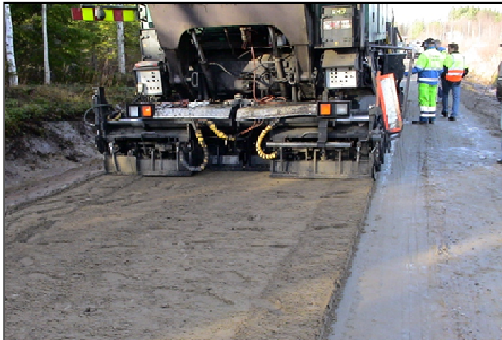
Stabilising treatment of base course materials
