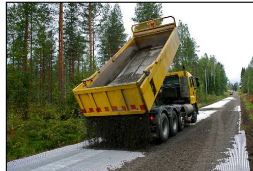
Applying basecourse on geogrid
