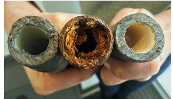
A lead pipe, a corroded pipe, and a pipe with protective orthophosphate coating. Photo: USEPA
