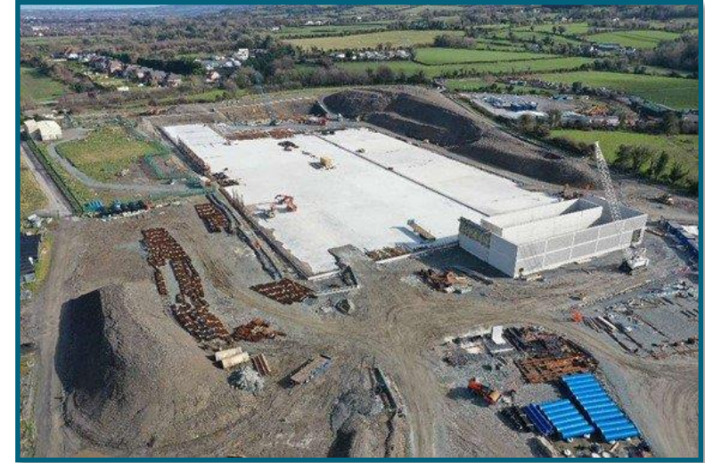
Photo: Saggart Covered Reservoir, from Uisce Éireann
