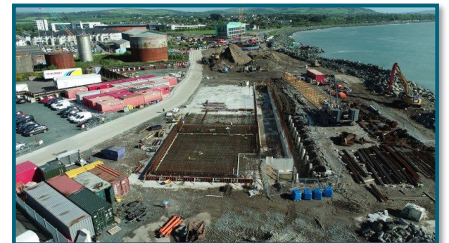
Photo: Construction of Arklow Waste Water Treatment Plant, from Uisce Éireann
