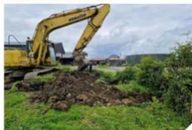
The willow bed is prepared by digging out an area 4 metres wide to allow for the sowing of the stems.
