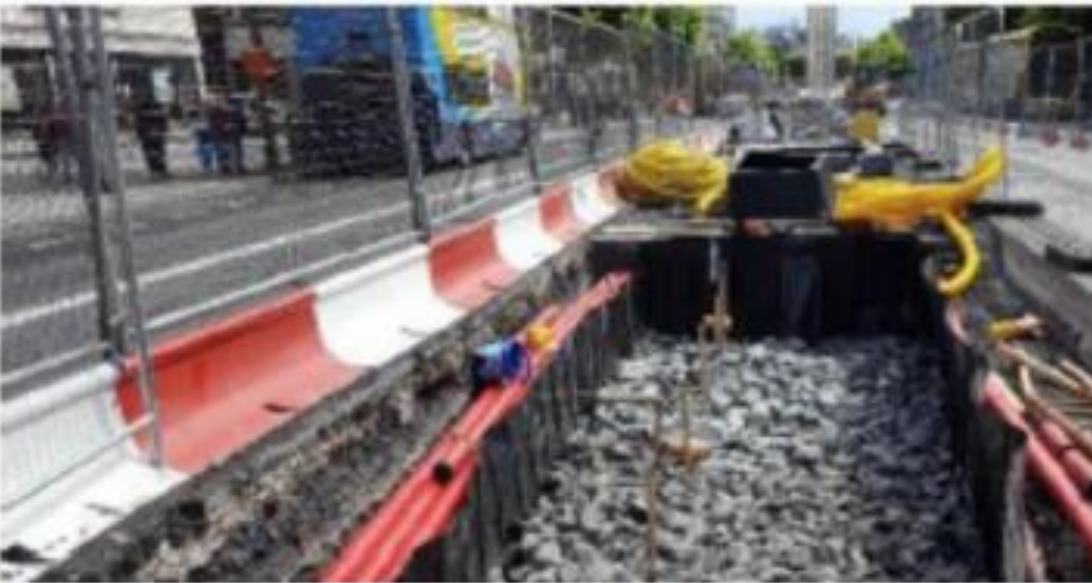
Figure 25 Stockholm tree pit system under construction in O'Connell Street
