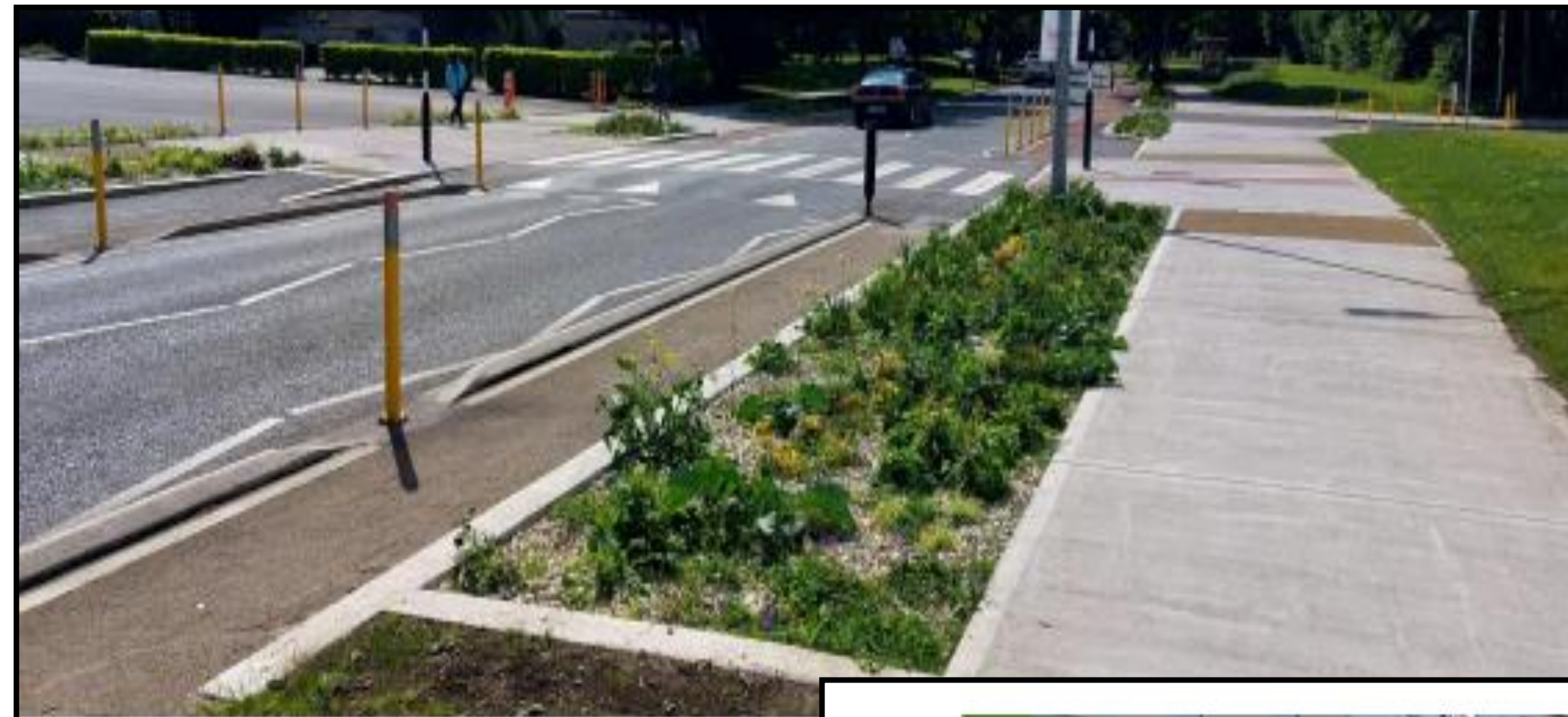
Figure 17 Rain gardens installed in existing verge, footpath width
