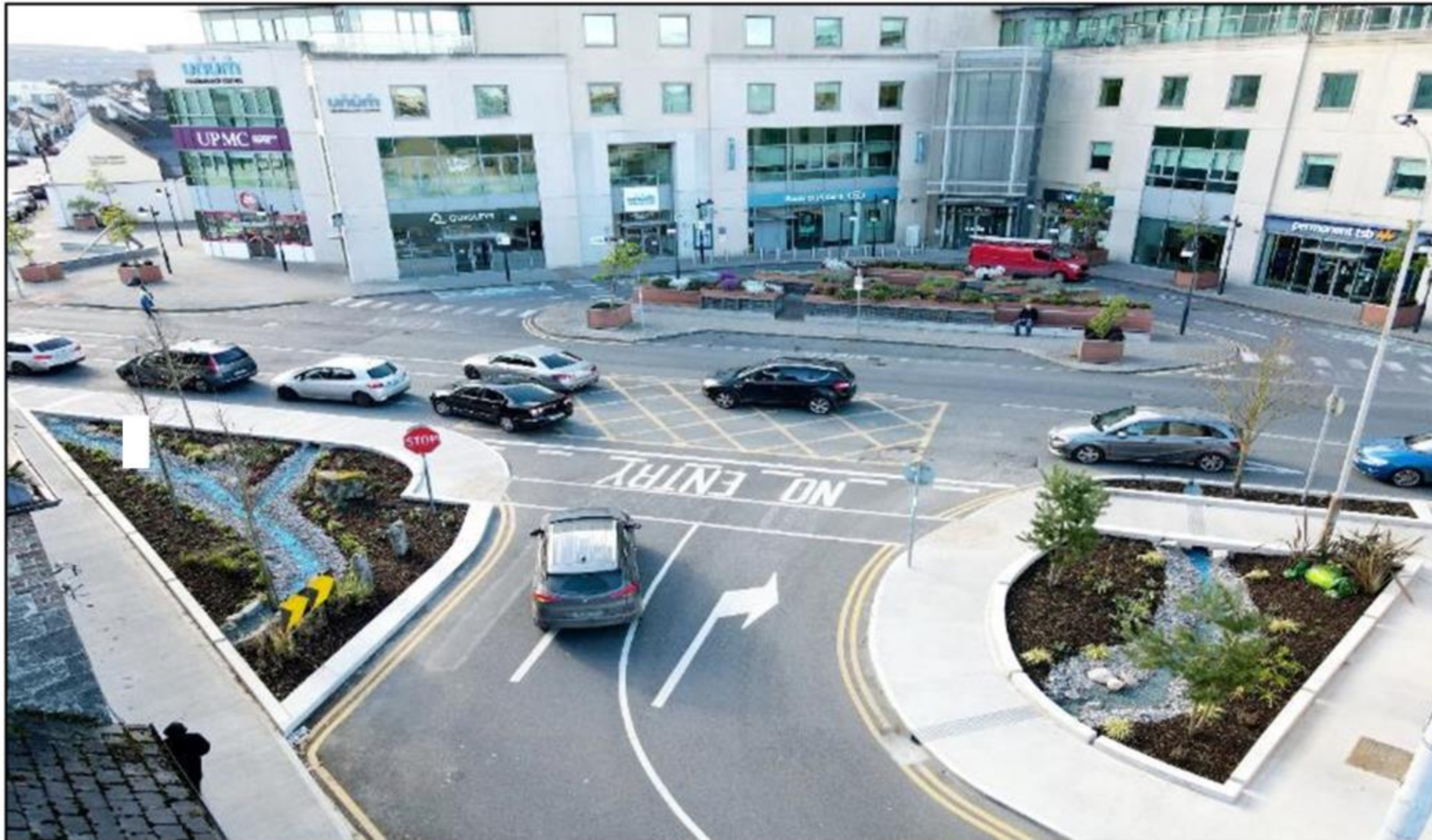
Bioretention Areas (Rain Gardens) – Pollerton Road/Green Lane Junction
