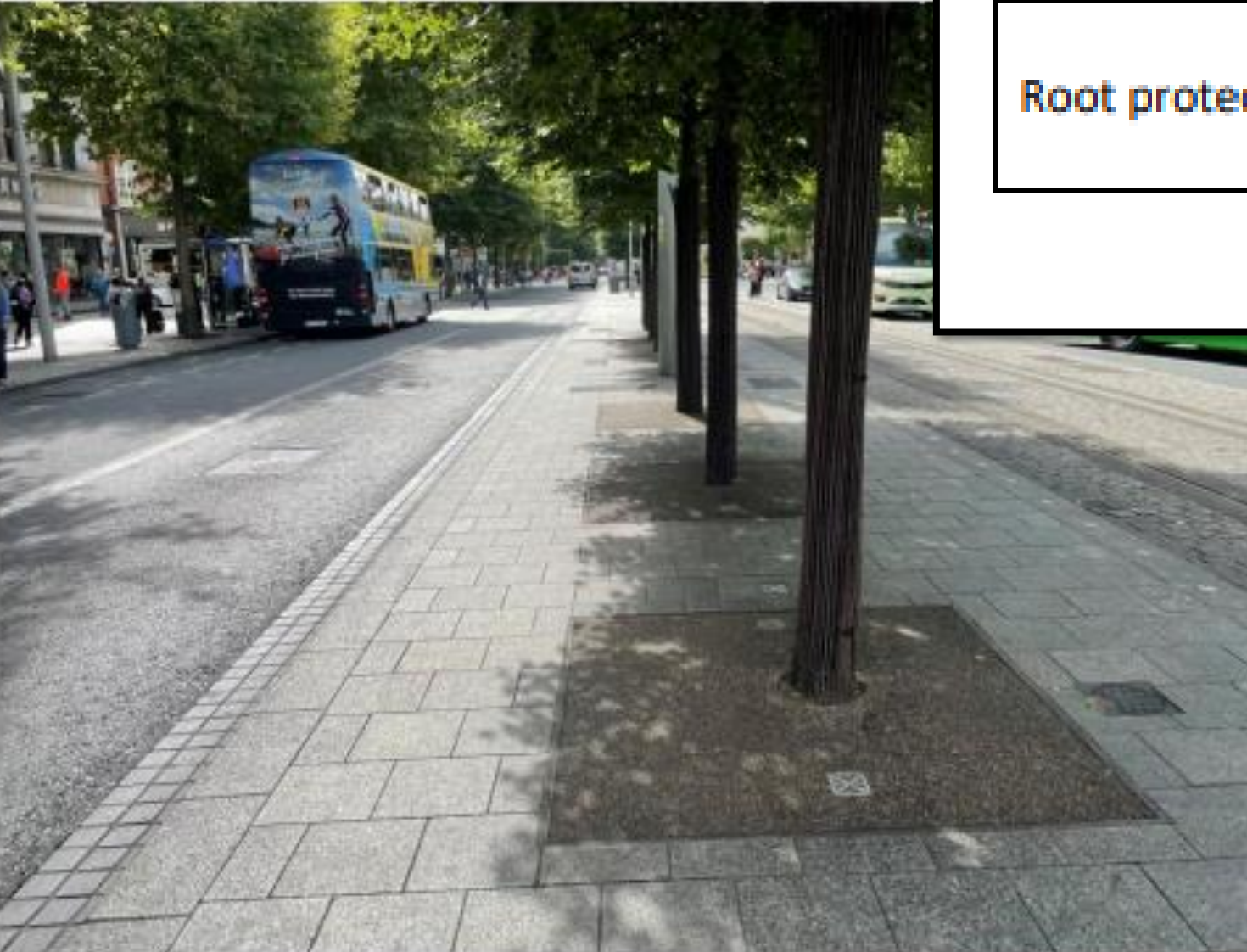
Figure 26 Completed scheme for the Stockholm tree pit system in O'Connell Street Dublin
