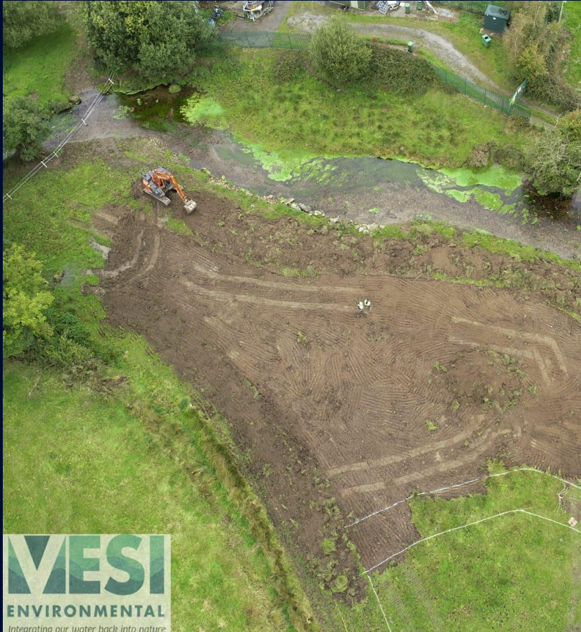
General Site Clearance Completed
