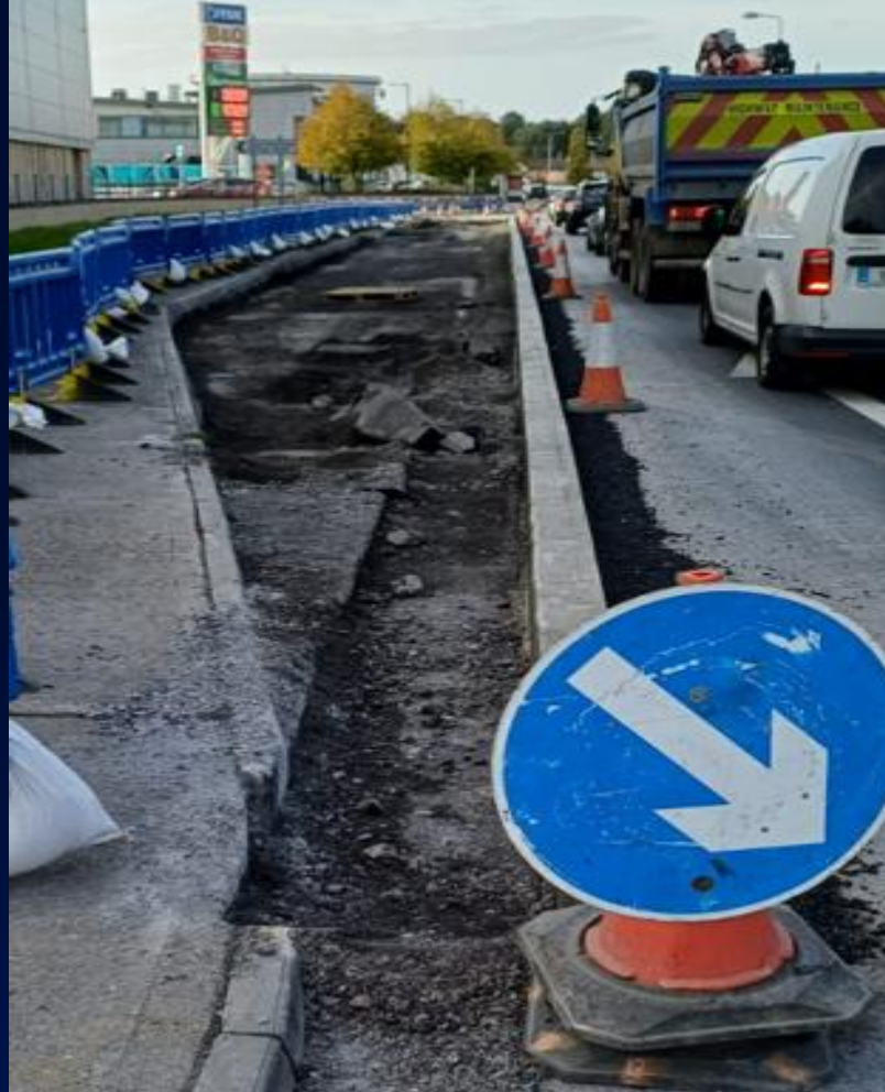
Excavation commenced Kerb Installed
