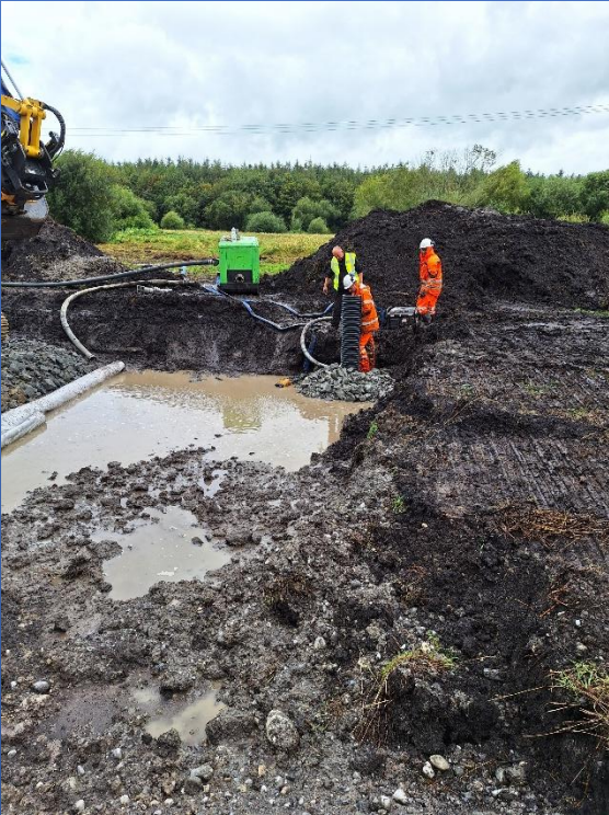
Photo 1: Keep the sump close to the front of the excavation
