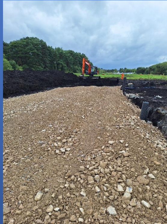
Photo 3: Sumps left in fill if required later.
