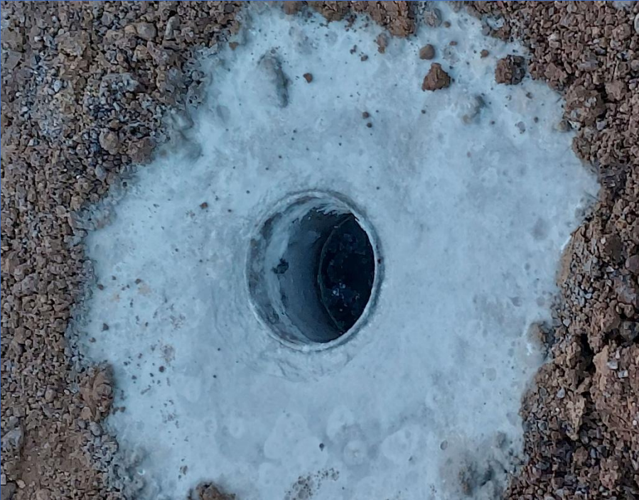
Steel Liner in Concrete
